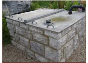
Concealed pump backs waterfall
